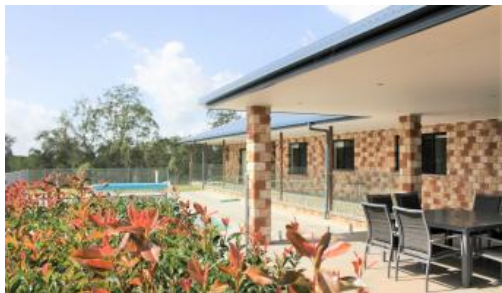
320A McDonald's Bridge Road, Kyogle
